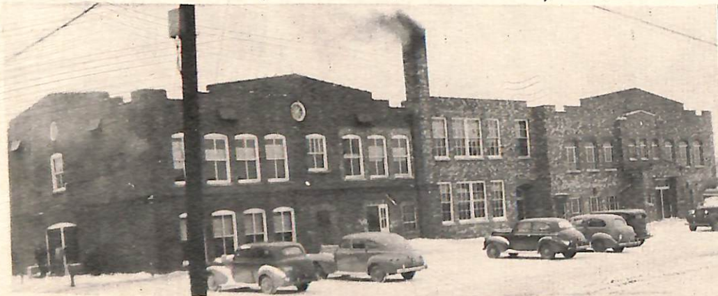
THE MODERN LINCOLN HIGH SCHOOL BUILDING Moberly, Mo.
